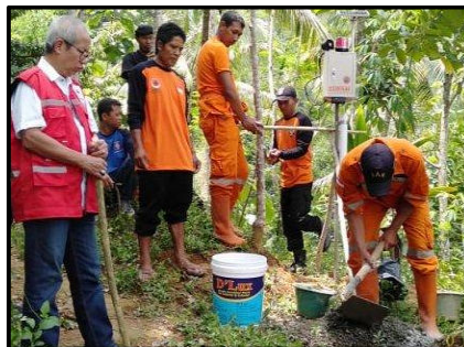
Gambar 5 Pemasangan Early Warning System
