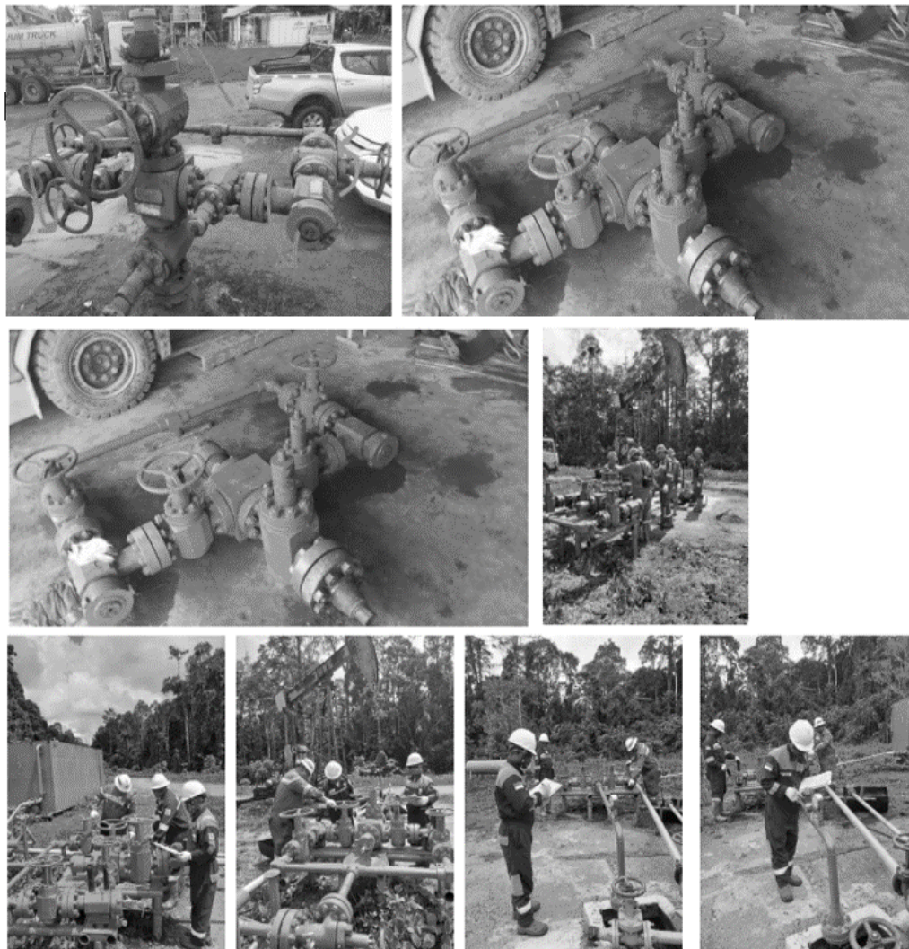
Figure 8. The Installation of Modified Choke Manifold in Simson well
