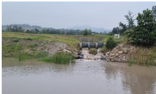
Figure 4. Illustration of check dam and riprap (rock)
