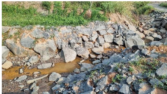
Figure 5. Illustration of Riprap (rock) in Drainage Channel
